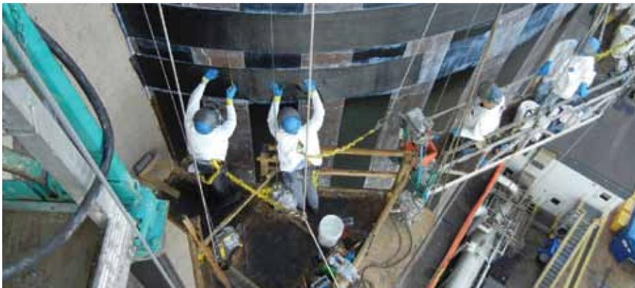
Installation of CFRP on an industrial silo.
