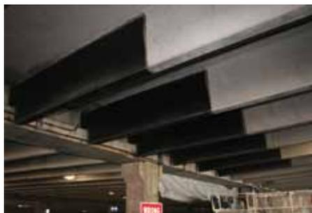
CFRP reinforcement on parking garage beams.
