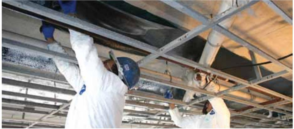
*Additional tension reinforcement increases the flexural strength of slabs when FRP is adhered to the tension side.*
