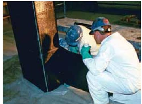
Wrapping FRP fabrics around columns increases the shear and axial strength to improve ductility and energy dissipation behavior.
